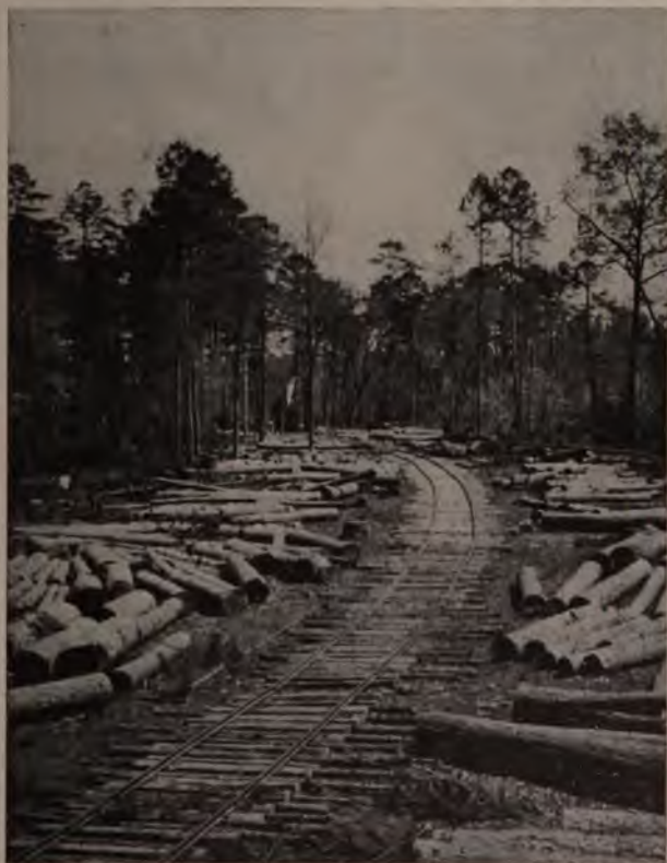
FIG. 80. — A Spur Logging Railroad corduroyed with Poles. Arkansas.
